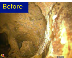
Underground video screen-grab showing collapse
