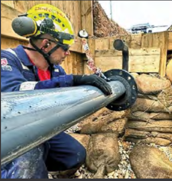
Rehabilitation of a hydrocarbon pipeline with around 200 bends
