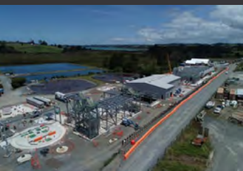
A bird's-eye view of Snells Beach Wastewater Treatment Plant
