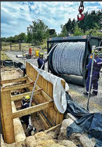
Rehabilitation of a hydrocarbon pipeline with around 200 bends
